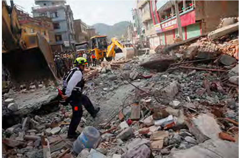
An unnamed USAID rescue worker inspects the site of a building that collapsed in the 25 April, 2015 earthquake in Kathmandu, Nepal, on May 12, 2015. Credit: Niranjana Shrestha, Associated Press.
